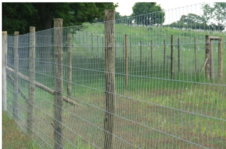
Photo 2-14: Typical deer security fence
